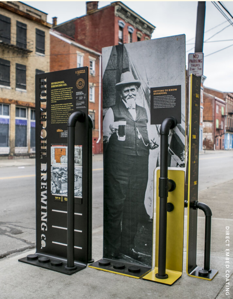
Fig. 4. This marker along the Brewing Heritage Trail in Cincinnati, Ohio, was produced with powder-coated graphics on a steel structure.
