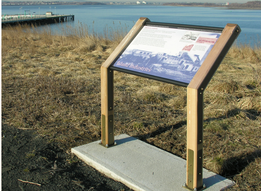
Fig. 14. At Boston Harbor Islands National & State Park, a cedar-frame structure with brass fittings supports a sloped interpretive panel.
